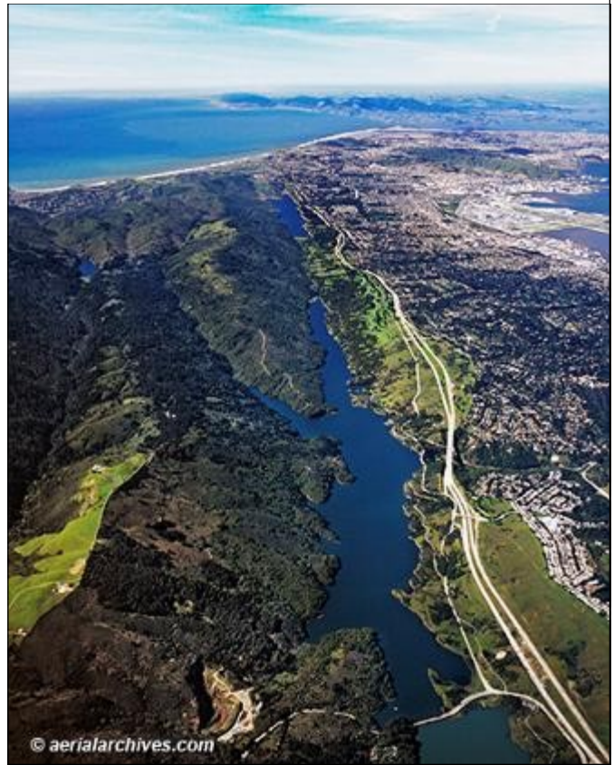
Lower Crystal Springs Lake. On the east is I-280. Highway 92, the main roadway through the mountains, crosses the dam between the two reservoirs. Courtesy © Herb Lingl/aerialarchives.com.
