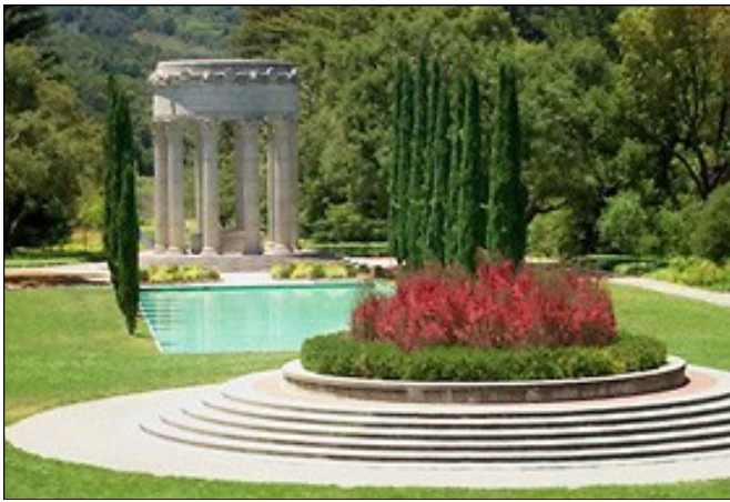
The Pulgas Water Temple, a stone pavilion, was erected close to the Crystal Springs reservoir to celebrate the “mingling of the waters—when water brought from the Yosemite’s Hetch Hetchy Dam began to arrive in the Peninsula’s greatly enlarged water-holding facilities. Photo: San Mateo County Division of Parks.
